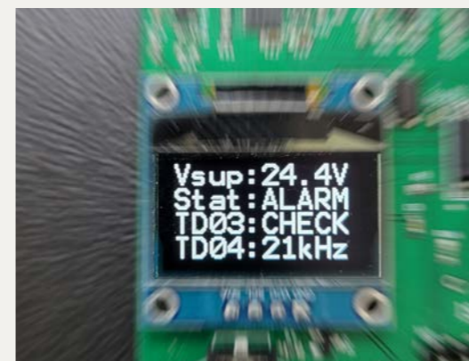
Check: transducer loose or corrosion
