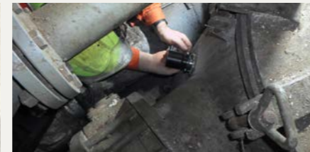
Installing transducer
