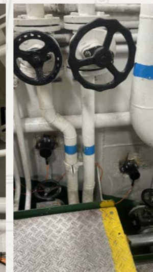
Transducers installed
